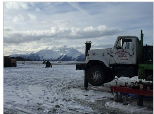
Exhibit 3-5: Wheaton Water Wells installs Test Well 2. Photo taken facing west.
